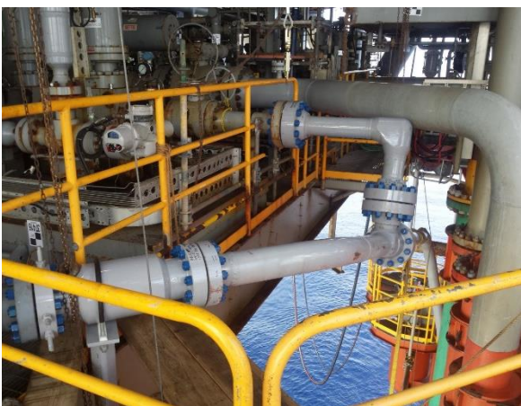
Figure 5. Post-Installation Piping Assembly.
