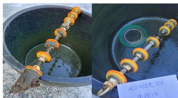
Figure 8. Pigging of downstream section. Left: Reference test. Right: Use of cold flow (seeding and robot), 0 % WC.
